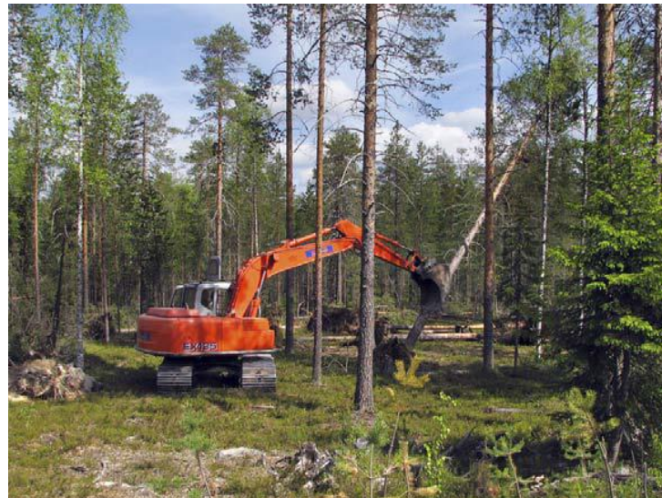
Pushing down with an excavator Photo: Juha Siekkinen
